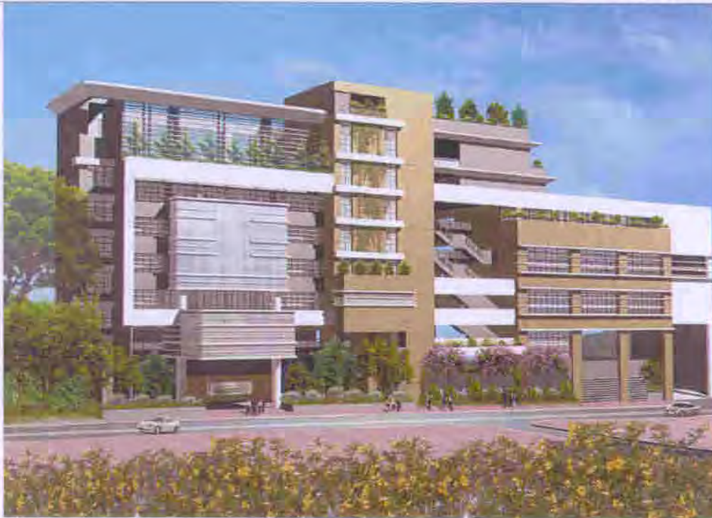
VIEW OF THE SCHOOL PREMISES FROM WESTERN DIRECTION (ARTIST'S IMPRESSION) 從西面望向校舍的構思圖
