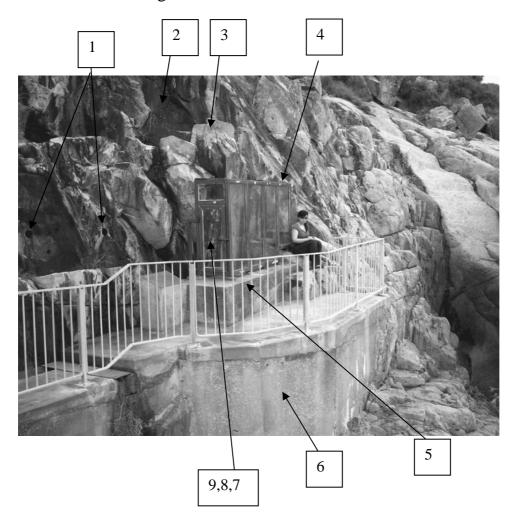
1. holes drilled for water drainage – unsightly and unknown impact on rock's internal hydrology
