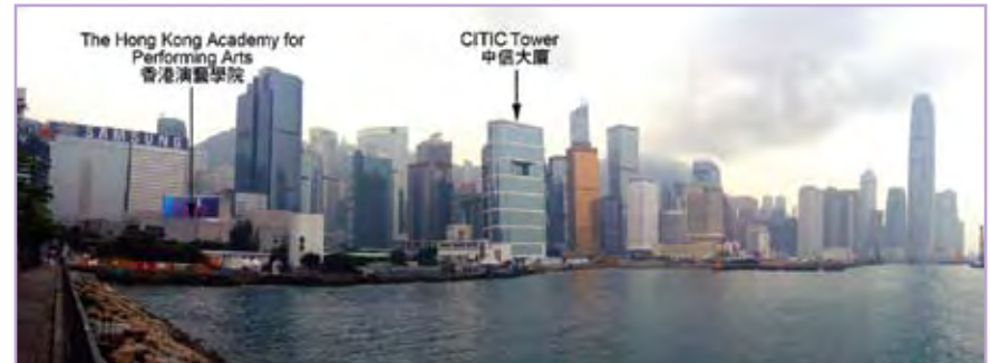
Sites 5 & 6 North of CITIC Tower and near HKCEC Extension
