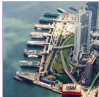
Site 1 near Central Piers No. 4 - 6
