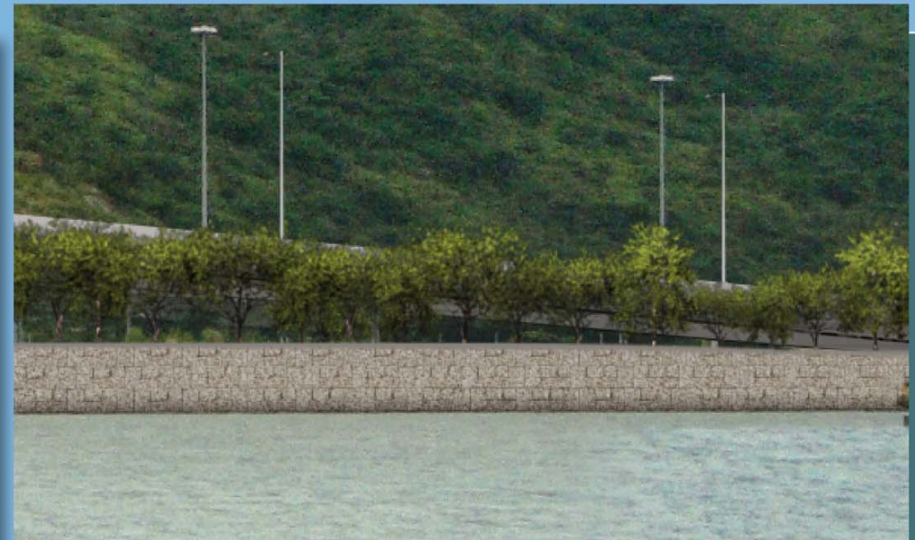
Elevation (Close-up View) of Proposed Project (Reclamation Scheme) 擬建計劃的特寫立面圖(填海方案)
