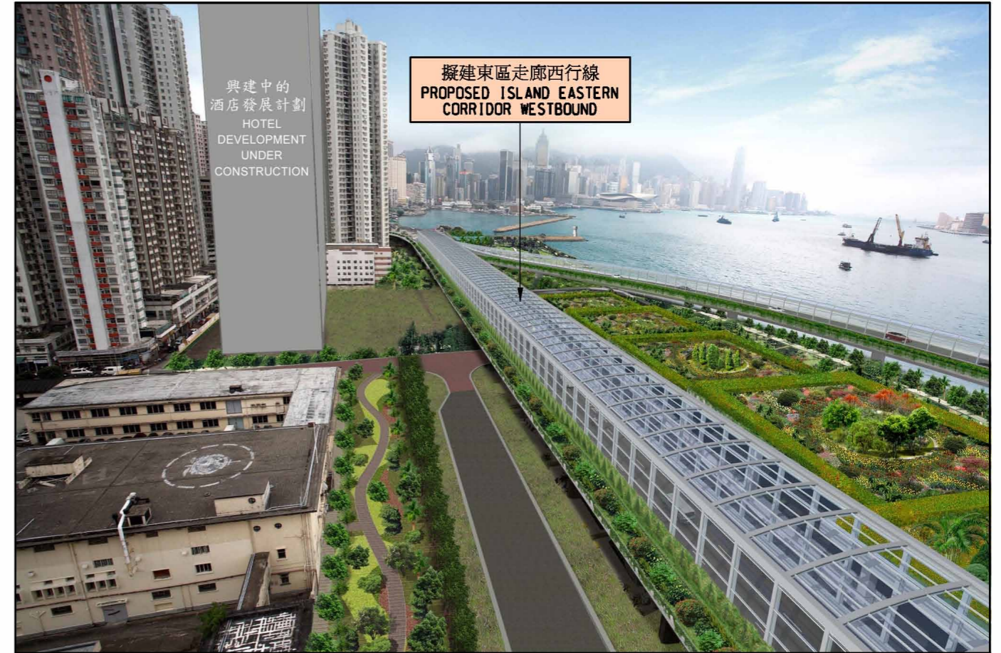
視圖 2 - 北角東區走廊的半開放式隔音罩 VIEW 2 - NOISE SEMI-ENCLOSURES AT ISLAND EASTERN CORRIDOR AT NORTH POINT
