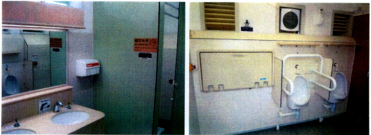
廁所改善後之內貌 INTERIOR VIEW OF TOILET AFTER IMPROVEMENT
