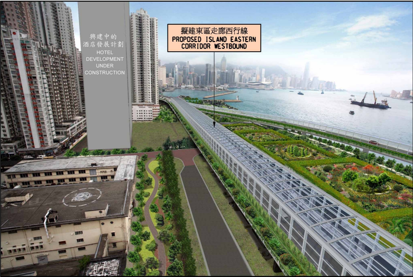
視圖 2 - 北角東區走廊的半開放式隔音罩 VIEW 2 - NOISE SEMI-ENCLOSURES AT ISLAND EASTERN CORRIDOR AT NORTH POINT
