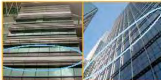
Use of shading devices – fixed or movable, located inside or outside the glazing, can control direct or indirect solar gain
