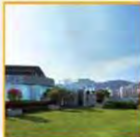
Rooftop greening reduces heat absorbed by the roof
