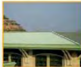
Non-absorbing roofing – roof covered by light-coloured or reflective membranes – absorbs less heat
