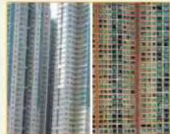
Wall-like barriers causing negative visual impact and reducing air flow
