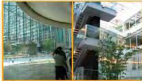
Enhanced use of daylight through building windows
