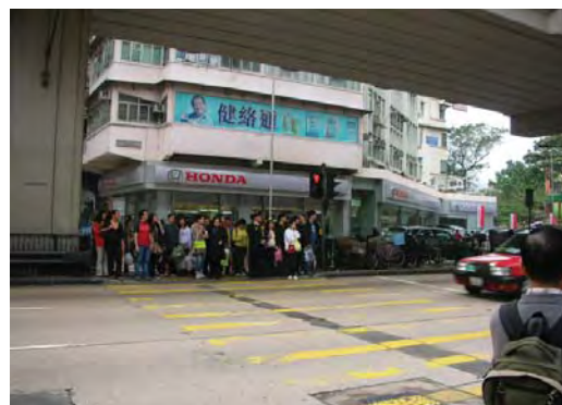
Existing Condition of Pedestrian Crossing at Prince Edward Road West 太子道西行人過路處現況
