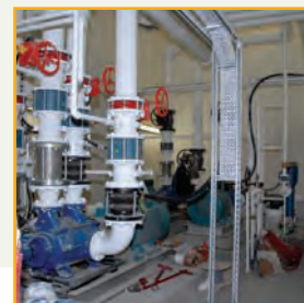
Sprinkler fixed & fire services booster pump room
