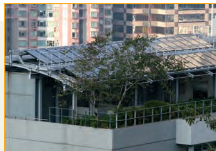
Rooftop solar photovoltaic panels can convert solar energy to electrical energy for the building
