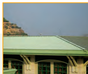
Non-absorbing roofing – roof covered by light-coloured or reflective membranes – absorbs less heat
