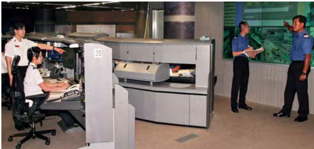
▼ Fire Services Communication Centre
