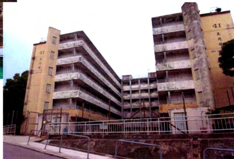
Existing Building 樓宇現貌
