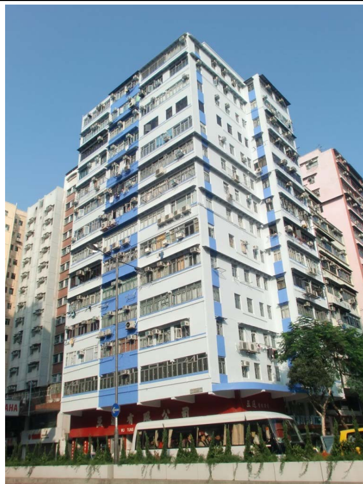
After repair works
