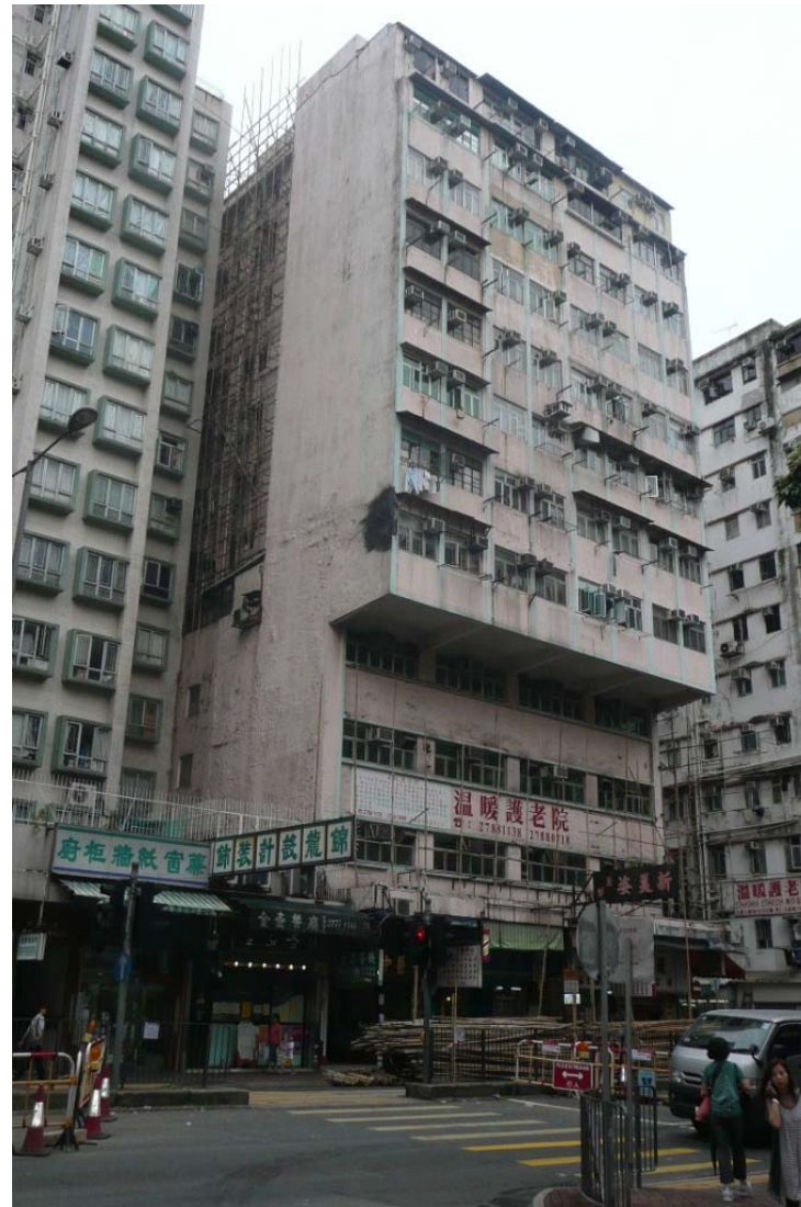
Before repair works
