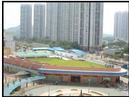
Grassed roof for commercial centre in Tin Ching Estate.
