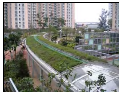
Covered walkway integrated with roof greening
