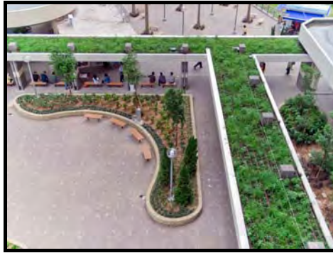
Covered walkway with roof greening in Upper Ngau Tau Kok Estate
