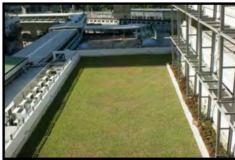
Grassed roof for commercial centre in Choi Ying Estate
