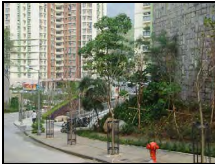
A line of trees planted along an estate road
