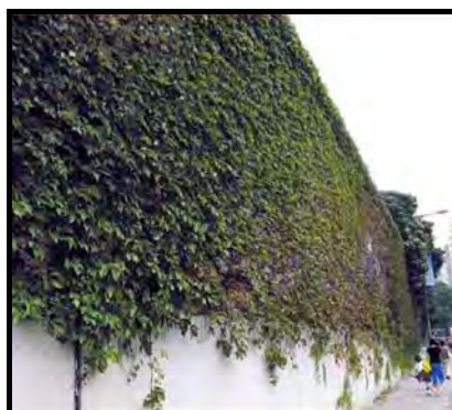
Greening by planting of climbers on a noise barrier wall in Kwai Chung Estate Phase 1
