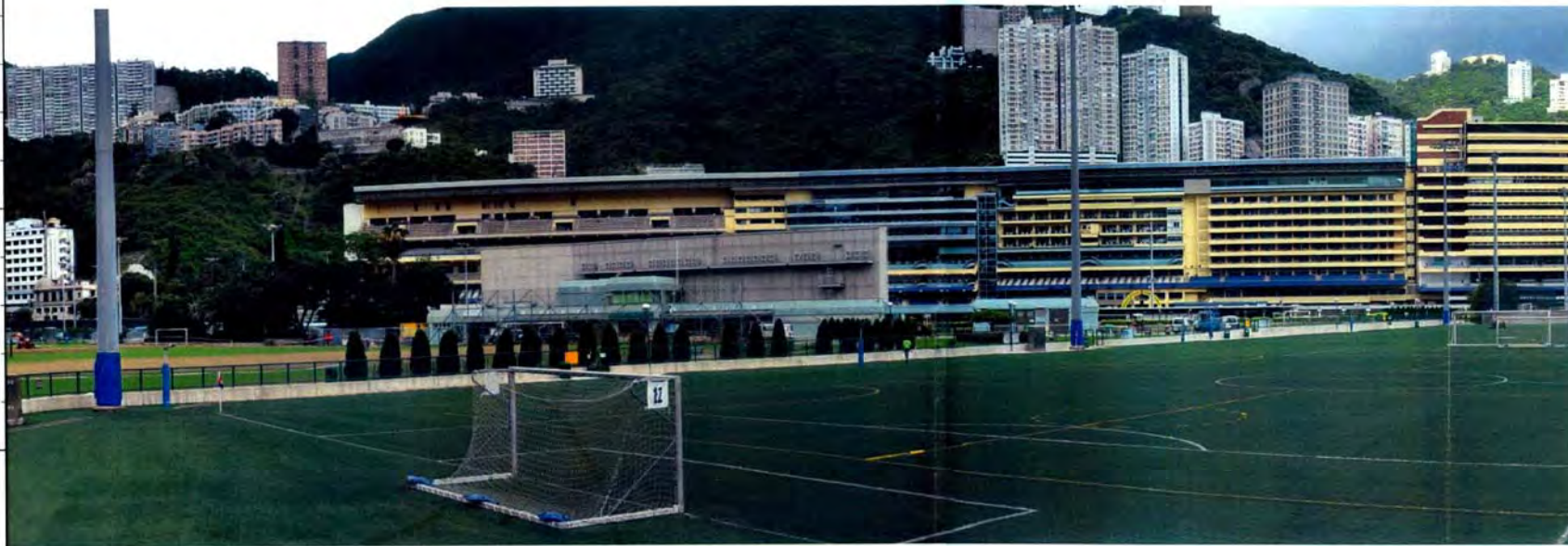
BEFORE CONSTRUCTION 施工前
