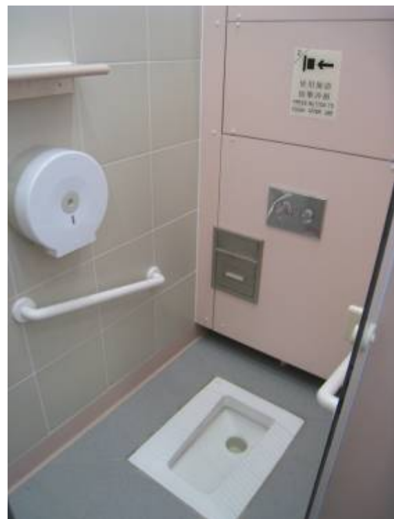
After conversion 改建後
