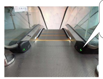
Energy saving escalator signal - the green arrow lighting signal indicates that the escalator is ready for use and its direction of travel.
