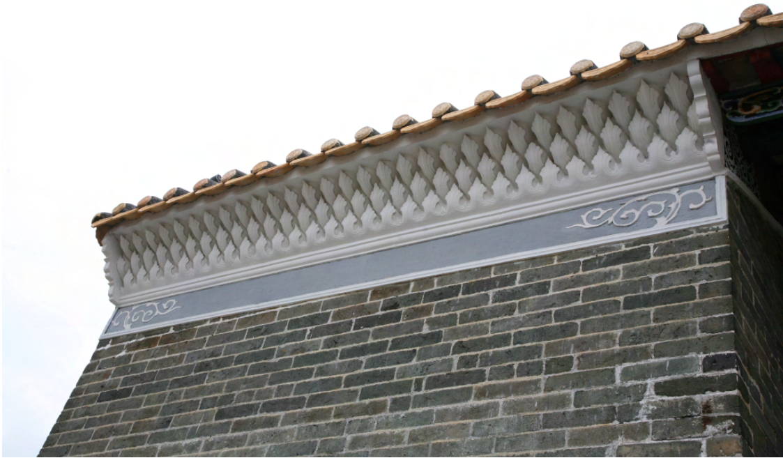
The plastered moulding under the eaves of the façade
