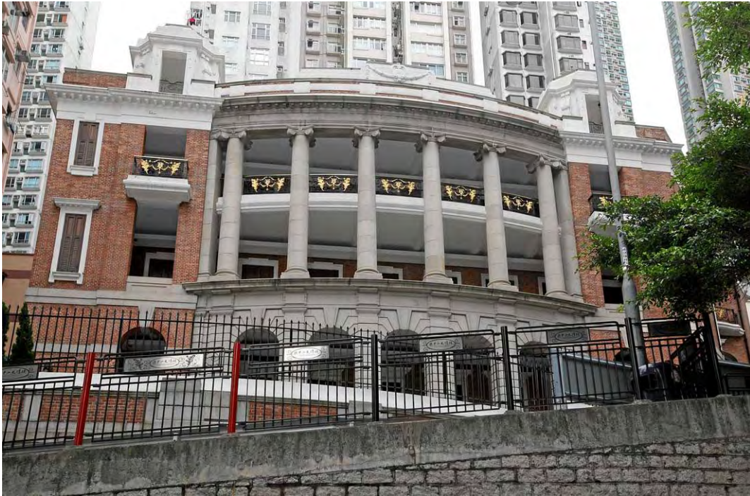
The front elevation of Kom Tong Hall facing Caine Road
