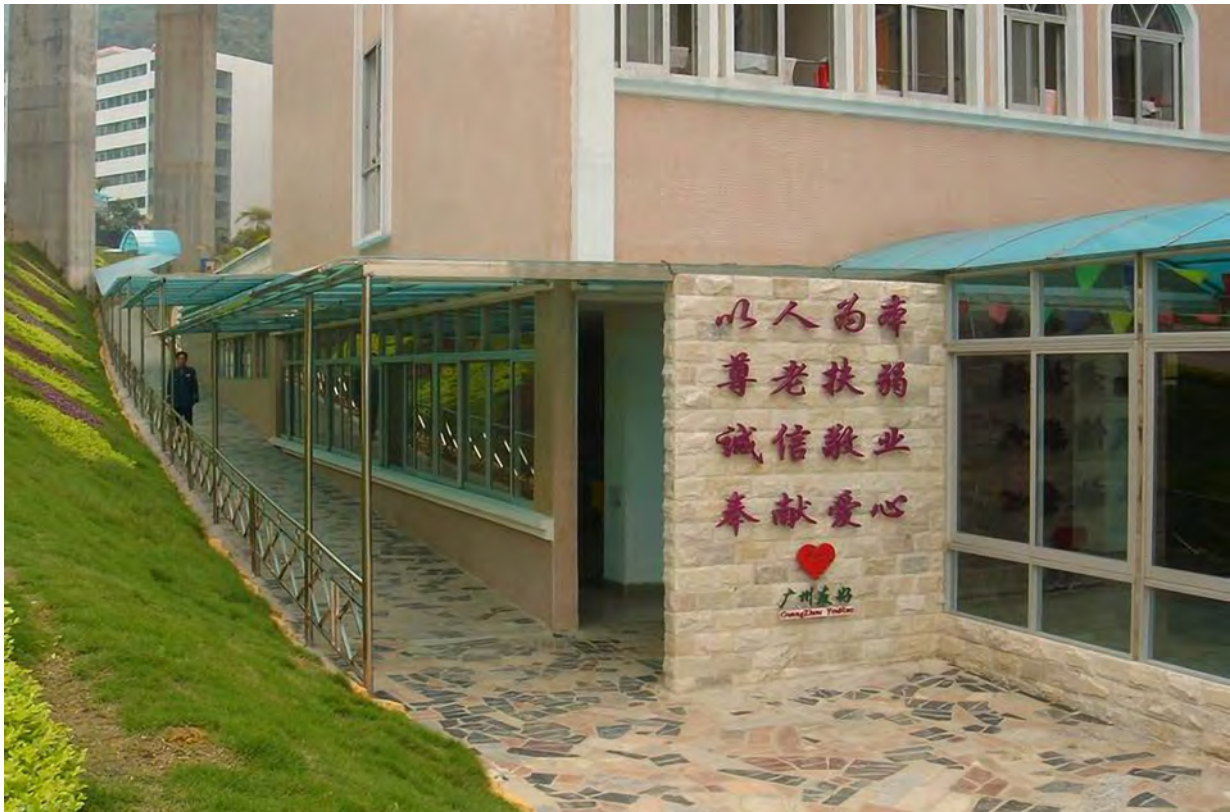
Figure 3-8 The Friendly Old Aged Home in Guangzhou: as more and more people choose a cross-boundary retirement life, there is a pressing need to provide quality social services for them.
