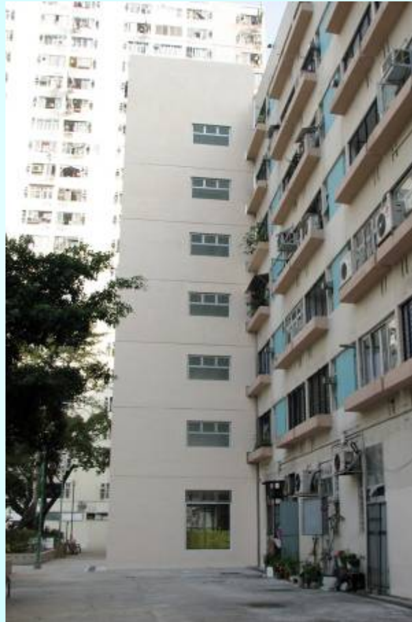
Completed – Lei Muk Shue (II) Estate (Block 4)
