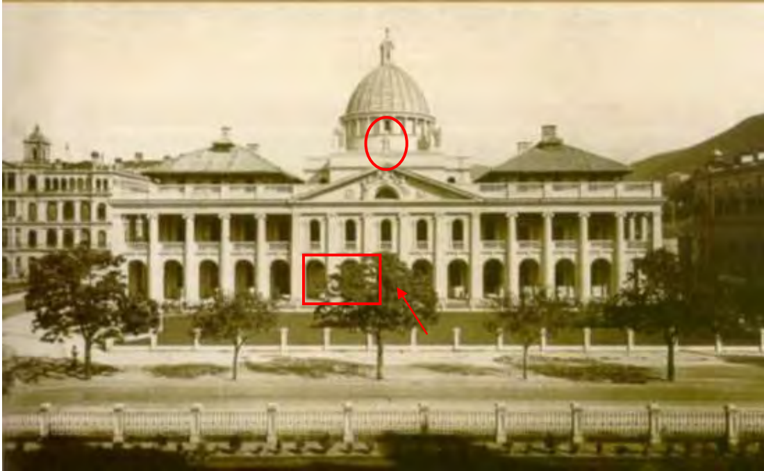
Fig. 43 The main elevation of the Old Supreme Court in 1915. The main entrance (pointed red) locating under the Statue of Justice (circled) signifies that all people are equally treated no matter what classes of these people are. The external windows of the cells (enclosed with rectangle) were originally designed with filled granite walls for security reasons which was matching with the details with 1899 design drawing. (Fig.44)
