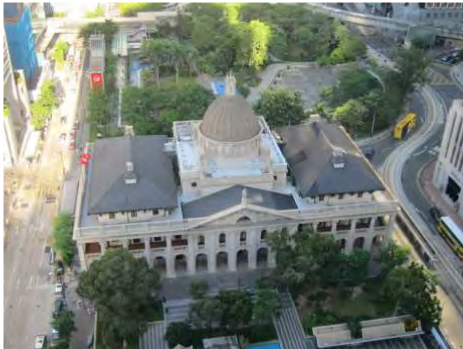
Fig. 35 Bird view of the roof level of the Old Supreme Court Building
