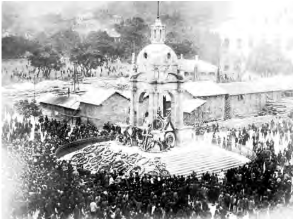
Fig.9 The condolence expression of Hong Kong citizens to the death of Queen Victoria in front of the Queen's Statue, 1901. Behind saw those straw sheds covering the foundation of the building with the pine tree trucks put beside which were ready for piling. (Source: Public Records Office, HKSAR)
