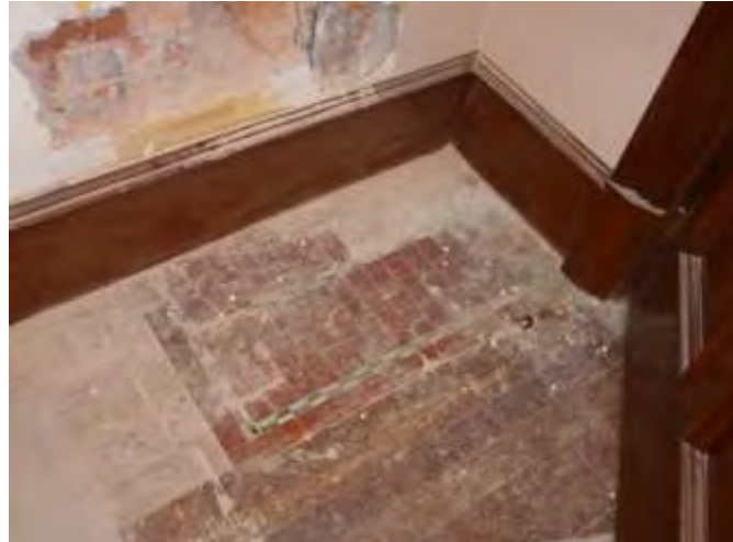
Fig. 80 (left) The exposed 2/F corridor. The existing tile surface is heavily damaged by later alteration works.
