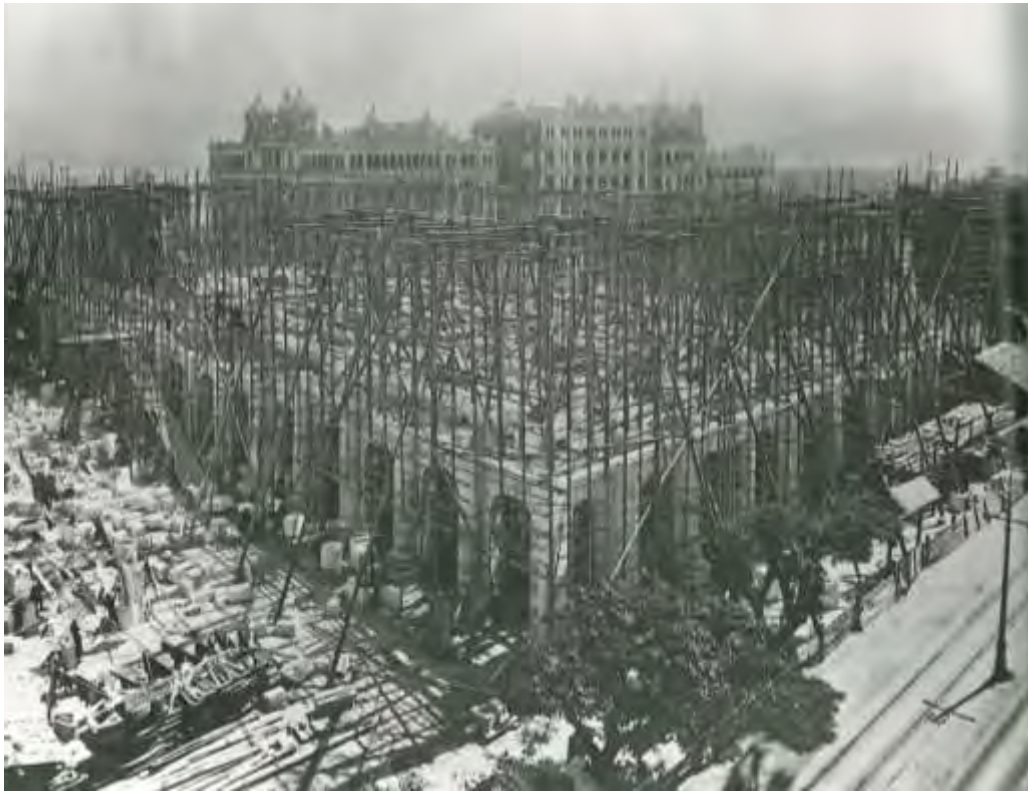
Fig. 10 The building of the superstructure, 1903 (Source: Hong Kong Museum of History)
