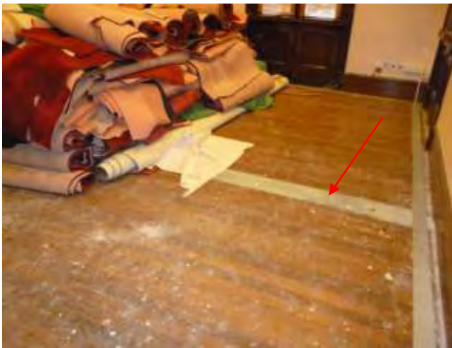
Fig. 73 (left) Pictures showing a room with original timber strip flooring. The floor was damaged by trunk work (pointed)
