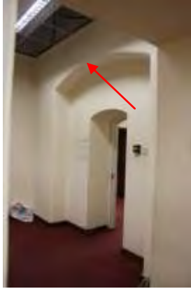
The original segmental arched opening of one of the cells (pointed)
