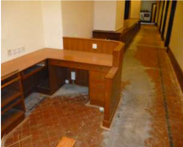
Fig. 80 (left) The exposed 2/F corridor. The existing tile surface is heavily damaged by later alteration works.
