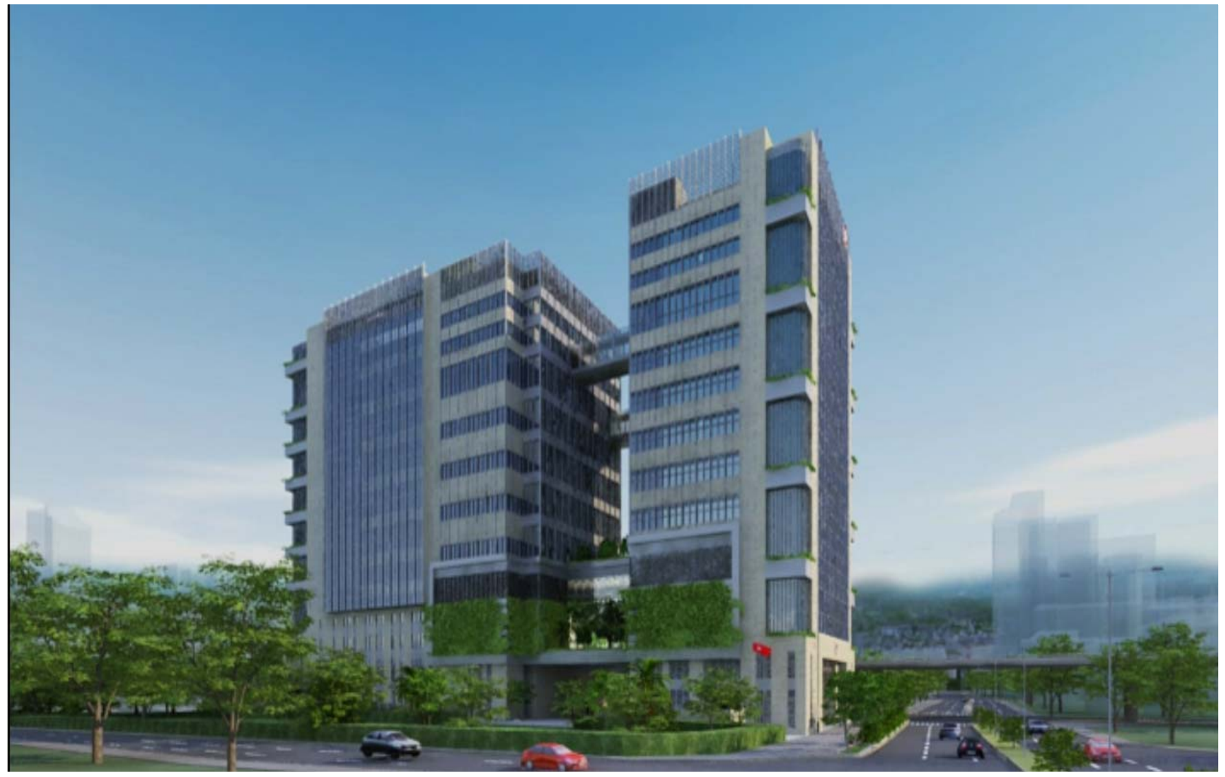
Building Image from Tonkin Street West
