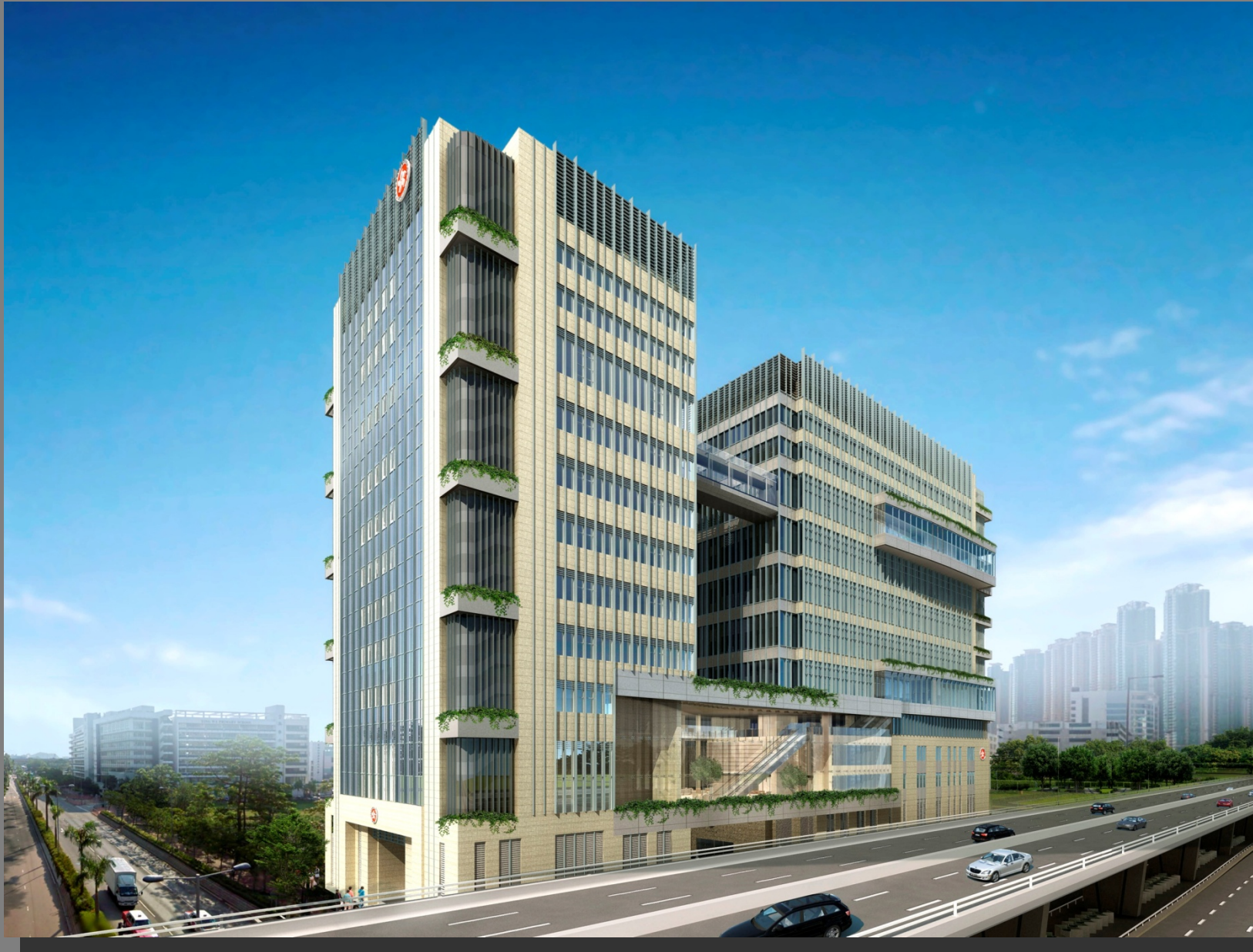
Building Image from West Kowloon Corridor
