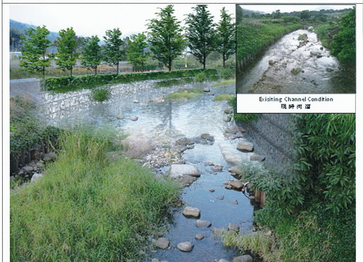
Photomontage of Upper Lam Tsuen River (after completion of works) 林村河上游的合成照片(竣工後)
