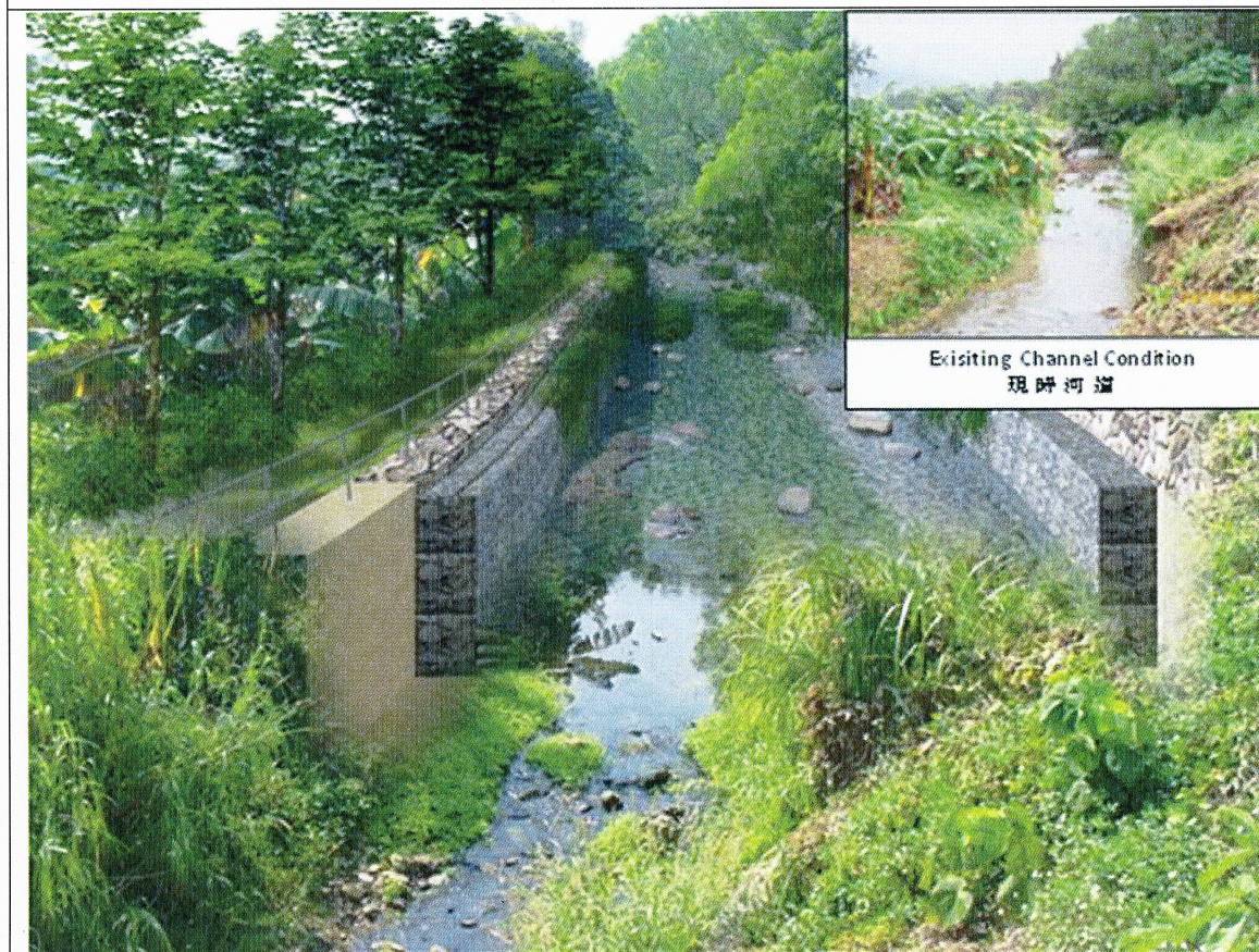
Photomontage of She Shan River (after completion of works) 社山河的合成照片(竣工後)
