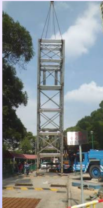
Pre-fabricated steel lift tower and footbridge – Cheung Ching
