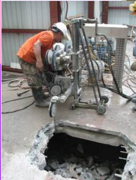
Diamond Wire Cutting
