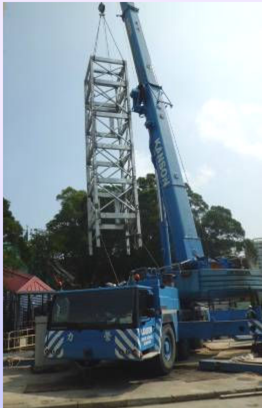
Pre-fabricated steel lift tower and footbridge – Cheung Ching
