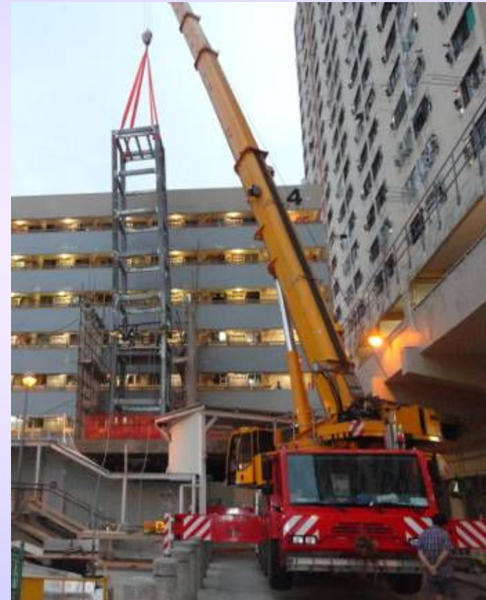
Pre-fabricated lift tower
