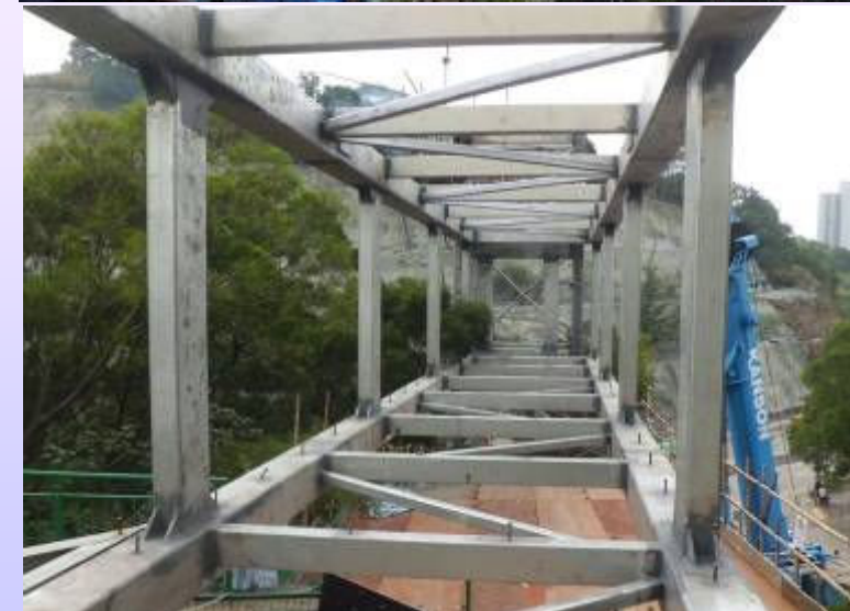
Pre-fabricated steel lift tower and footbridge – Cheung Ching
