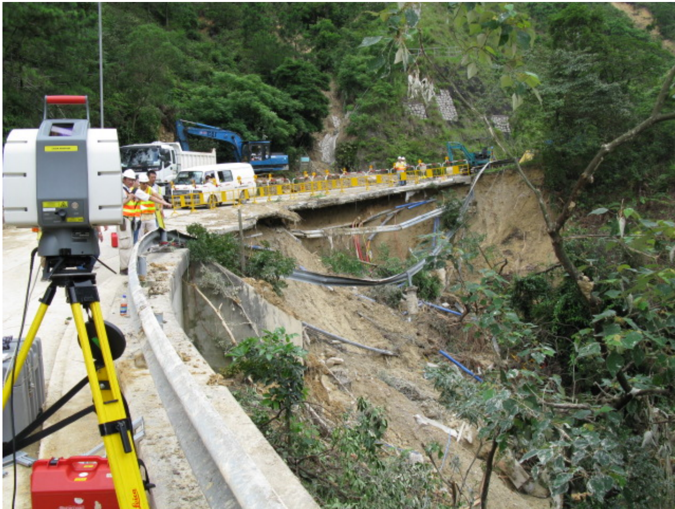
Figure 3 The Laser Scanner at Work on Keung Shan Road
