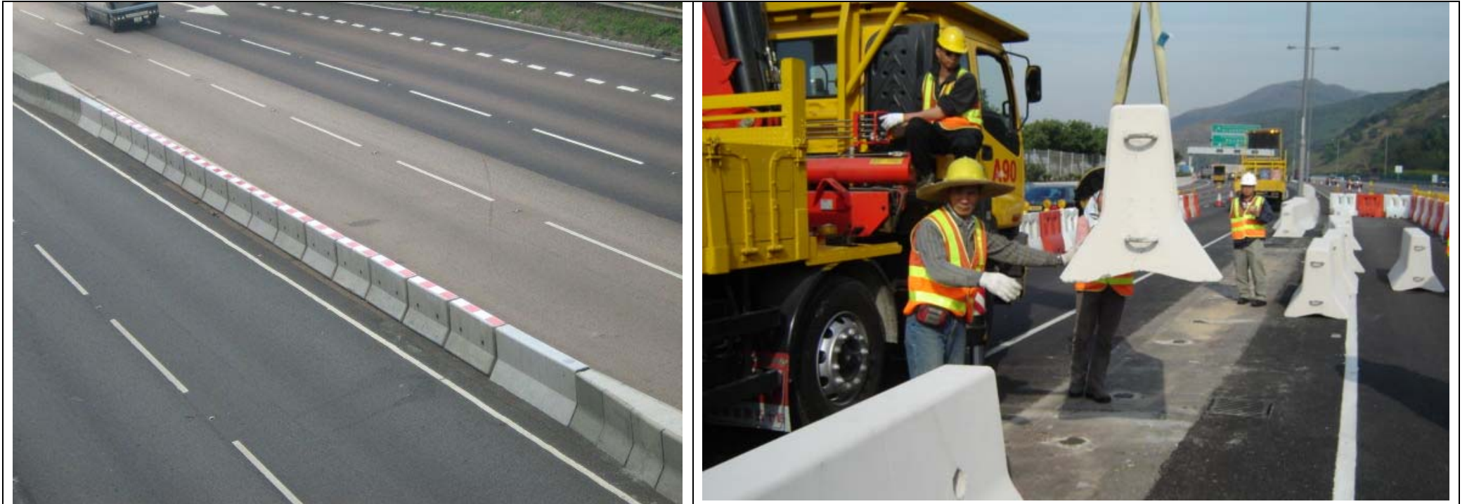
Figure 3: Removable Concrete Barriers
