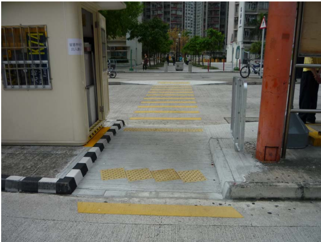
Figure 2 – Photos of Dropped Kerbs and Tactile Warning Strips
