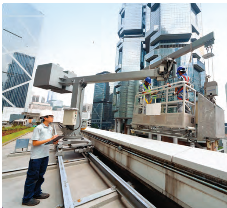
營運基金定期檢查高等法院吊船系統，確保系統安全及可靠運作。 EMSTF conducts regular checks to ensure the safety and reliability of the suspended working platform at the High Court.
