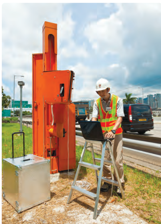
營運基金負責安裝及維修保養的雷達車速探測器有助監控車速，保障道路使用者安全。 EMSTF is responsible for the installation and maintenance of speed radar detectors, used to monitor vehicle speed and ensure the safety of road users.
