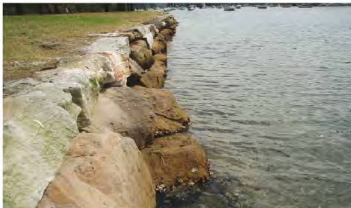
Figure 21: A seawall made from boulders of various size and shape with spaces between boulders providing sheltered habitat for organisms.
