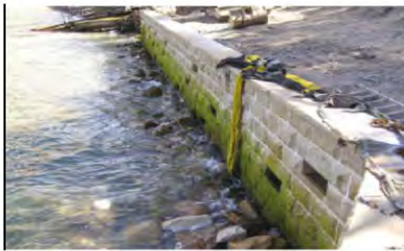
Figure 23: A seawall with blocks that extend outwards to create a varied surface, and cavities to provide sheltered intertidal-pool and subtidal-cave habitats for a variety of organisms.
