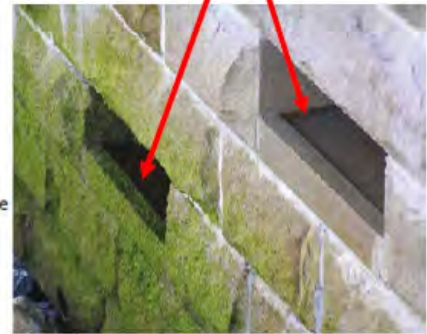
Figure 23: A seawall with blocks that extend outwards to create a varied surface, and cavities to provide sheltered intertidal-pool and subtidal-cave habitats for a variety of organisms.
