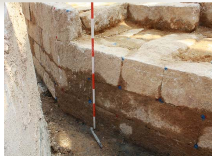
Close up view of seawall fragment 殘存海堤近攝
