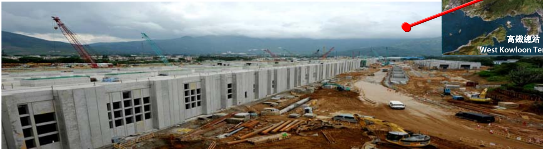
工地現況 Current status of works site
