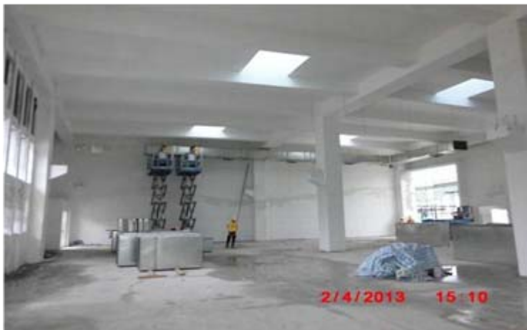
內部裝修及機電工程 Architectural builders works and E&M works
