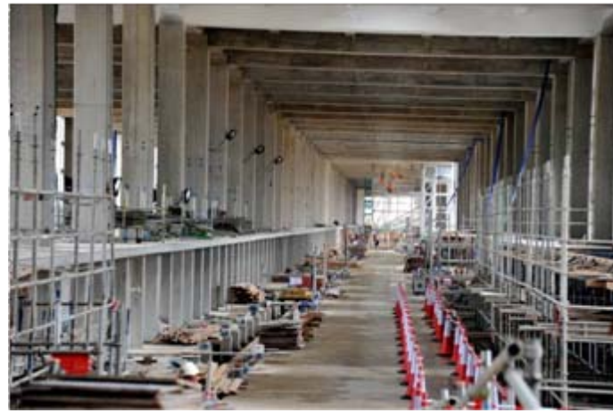
列車維修大樓內部 Internal view of Running Maintenance Shed
