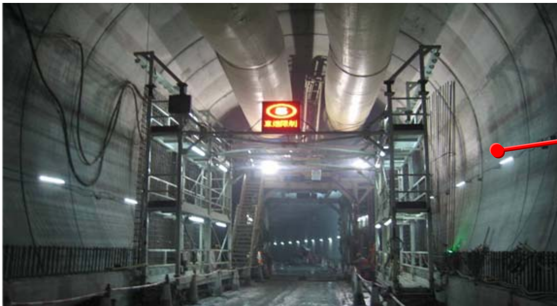
葵涌通風樓通風管道 Kwai Chung ventilation adit
