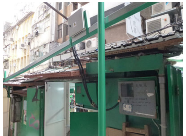
Figure 3.8.4 – Power Supplies From Overhead Cable Trunking System
