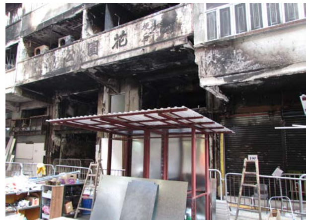
Figure 2.1.1 – Newly Erected Tin-sheeted Structure for Fixed Pitch Hawker Stall
