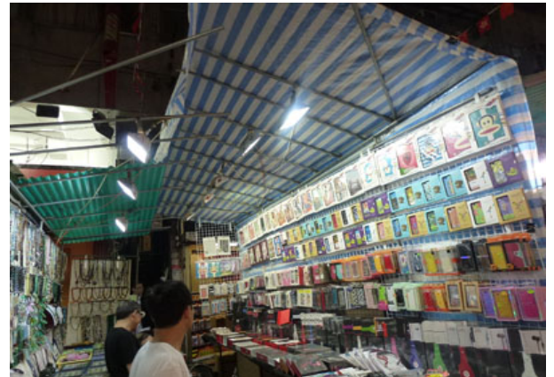
Figure 2.1.5 – Dismantable Hawker Stalls at Temple Street with Combustible Structures
