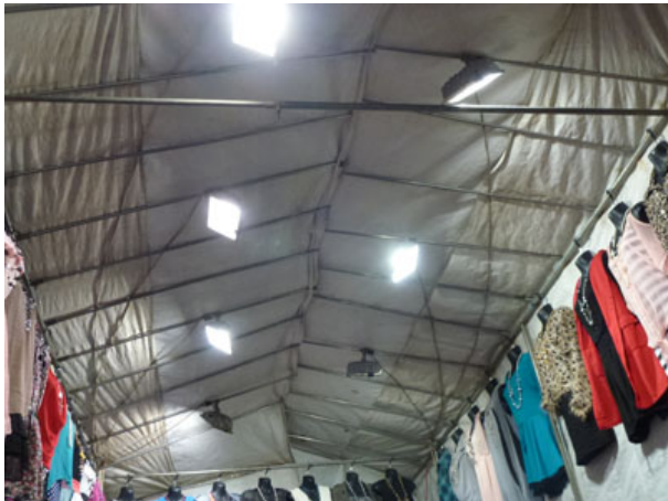
Figure 3.8.9 – High Power Consumption Halogen Lamps
