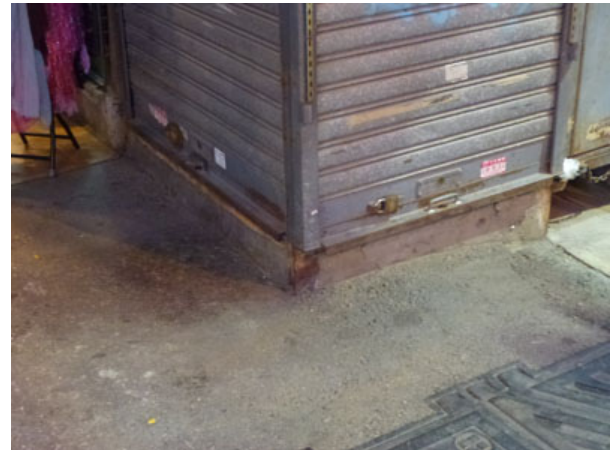
Figure 3.5.2 – Concrete Plinth Footing of Stall
