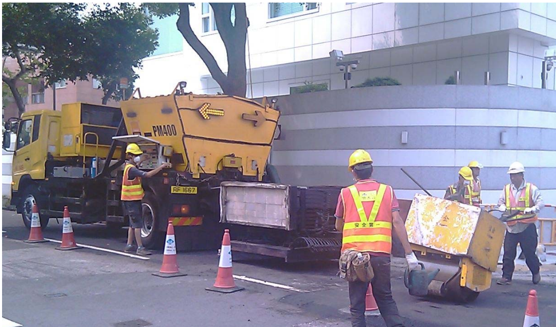
[Figure 3] Small-scale pavement resurfacing by thermal patcher
