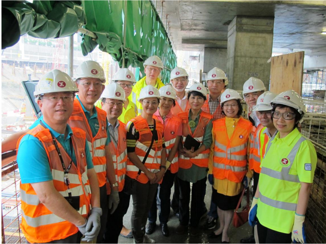
LegCo Members visit the construction site of the West Kowloon Terminus of the Hong Kong section of the XRL.
