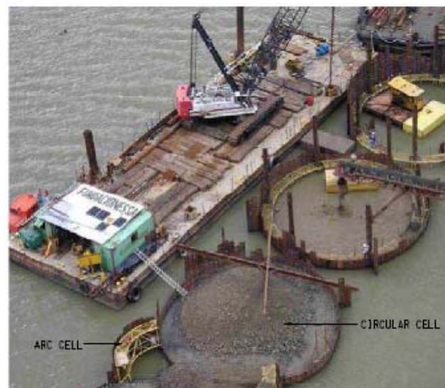
C. CONSTRUCTION OF ARC CELL CONNECTING TWO CIRCULAR CELLS
