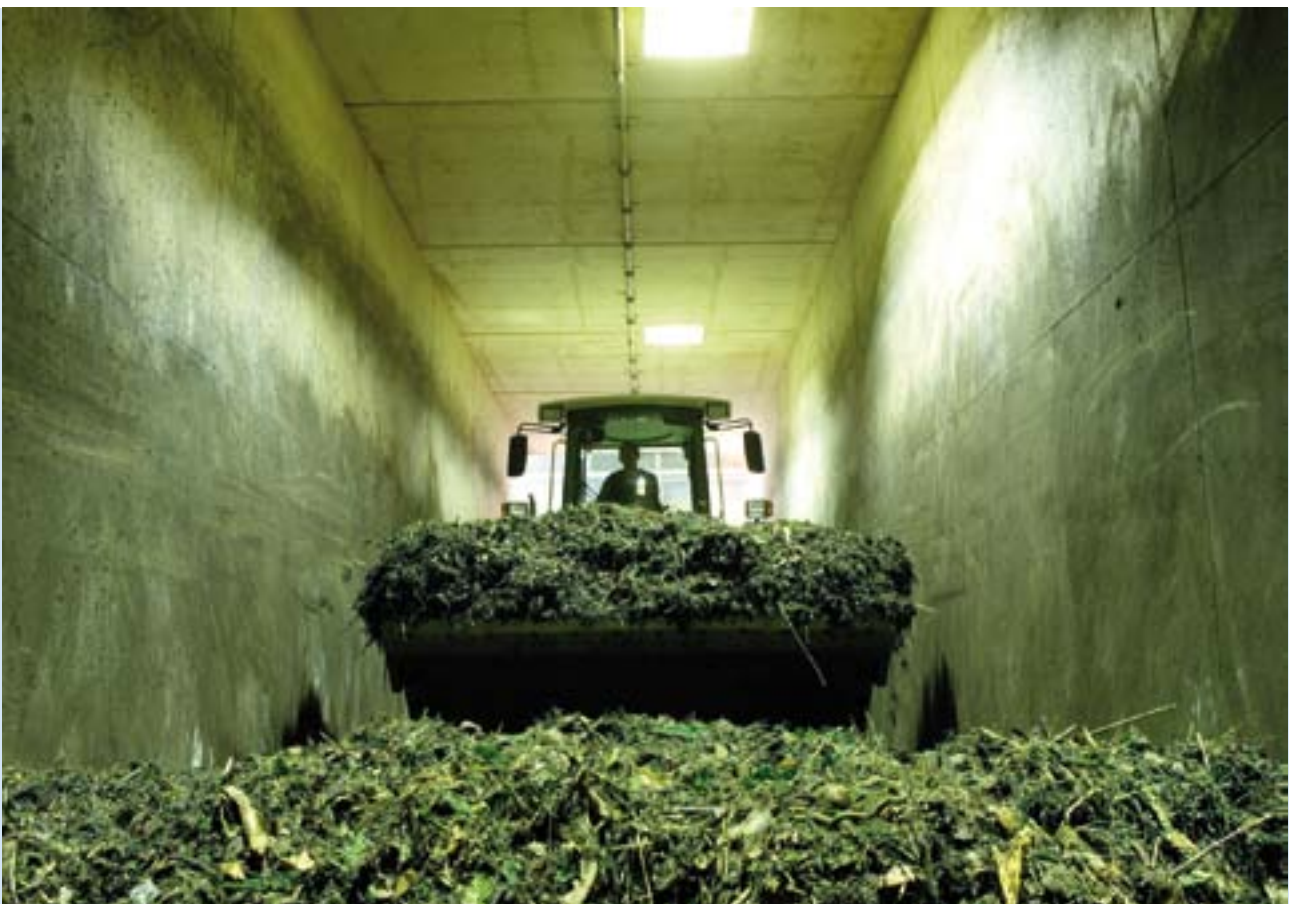
Rotting tunnel at a composting facility
