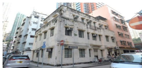
No. 12 School Street 書館街12號
