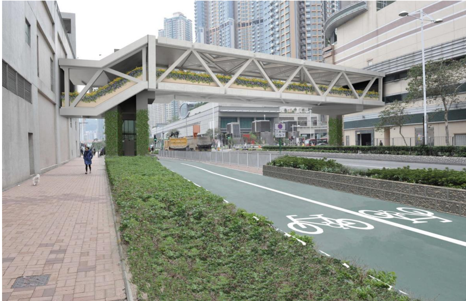
橫跨寶邑路連接將軍澳第55區及第65區行人天橋 Footbridge across Po Yap Road linking Tseung Kwan O Area 55 and Area 65
