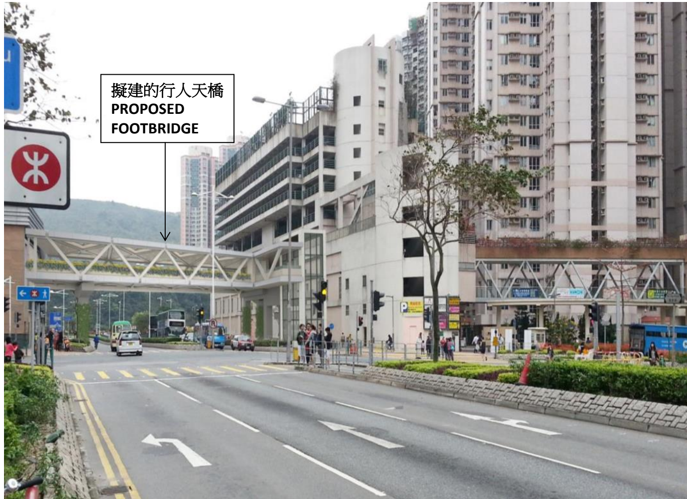
橫跨寶邑路連接將軍澳第55區及第65區行人天橋 Footbridge across Po Yap Road linking Tseung Kwan O Area 55 and Area 65
