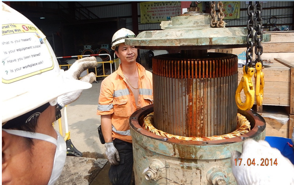
更換隧道鑽挖機鑽頭零件 Repair of TBM cutter motor
