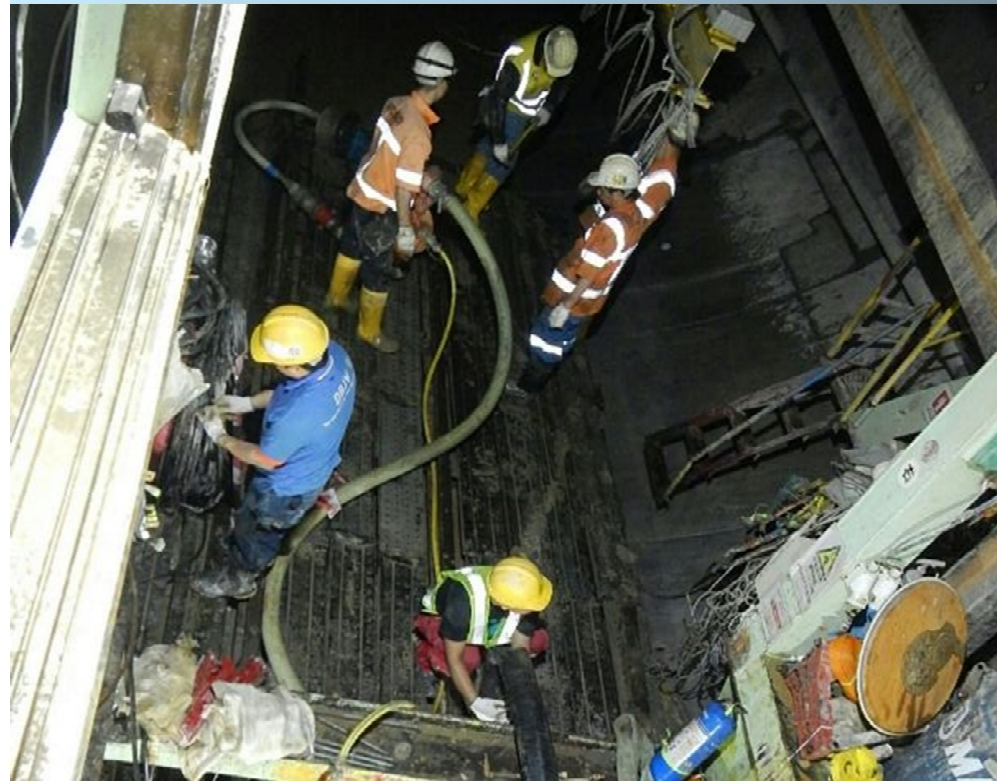
隧道鑽挖機清潔工作 Dewatering and cleaning of TBM
