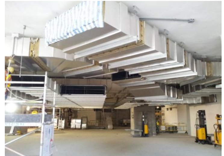
高鐵總站(南) – 屋宇設備安裝 WKT (South) – Building Services Installation
