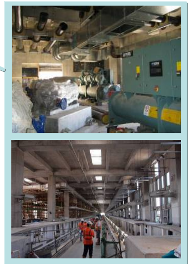
列車維修大樓內部 Internal view of Running Maintenance Shed
