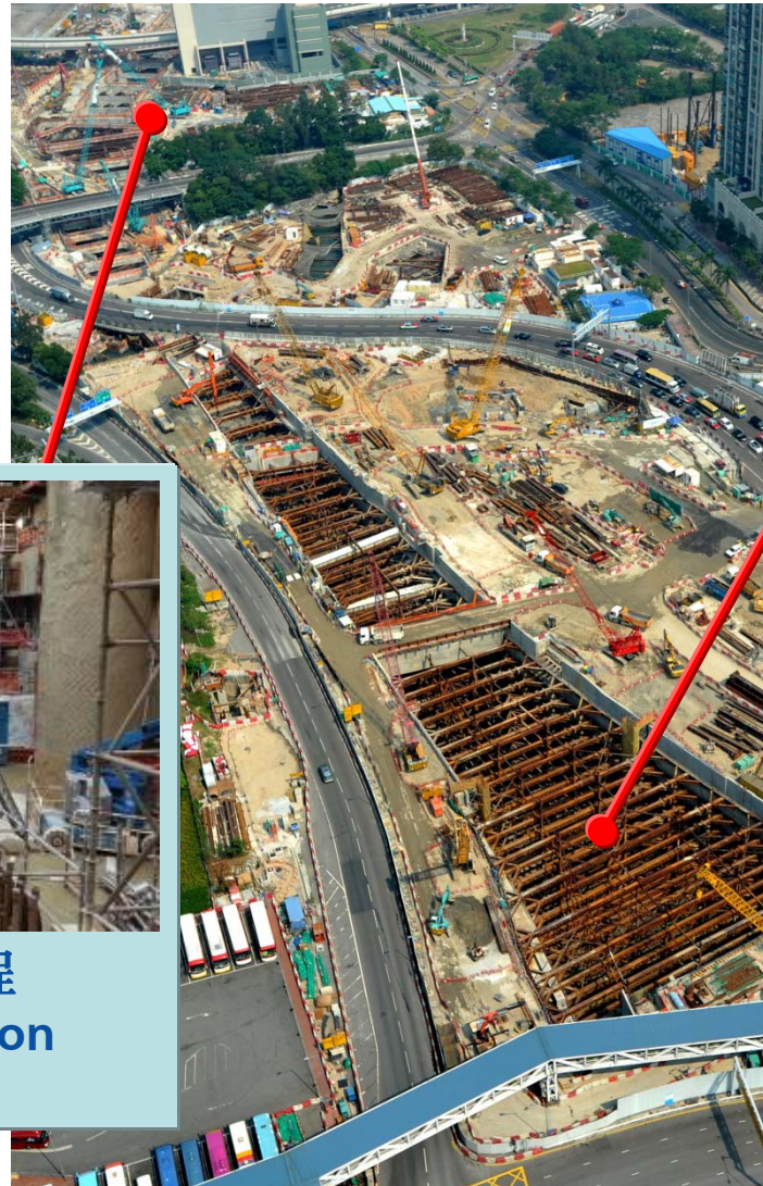
明挖隨填工程 Cut & Cover works
