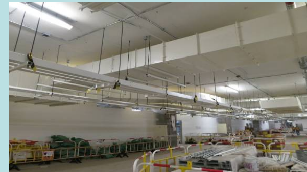
安裝風槽及電纜管道 Ductwork / Cable containment Installation
