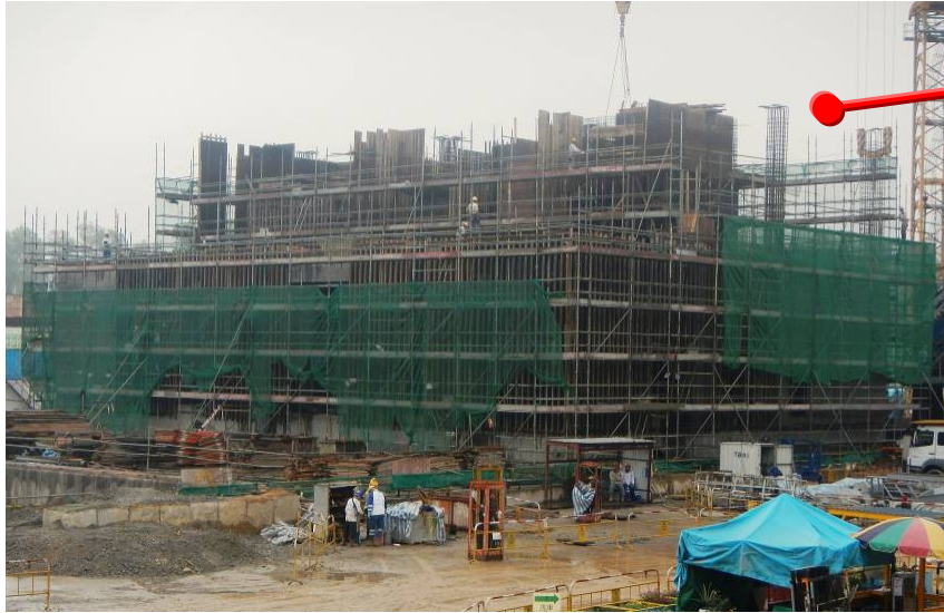
米埔通風樓之結構工程已大致完成 Structural construction for Mai Po Ventilation Building is substantially completed
