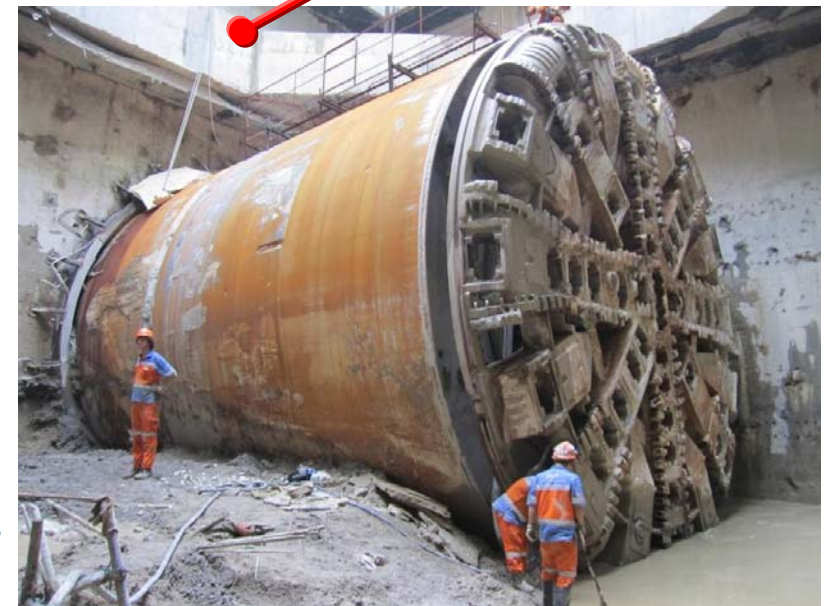
南昌以南的南行隧道於2013年9月貫通 Breakthrough of down-track tunnel at the south of Nam Cheong in September 2013
