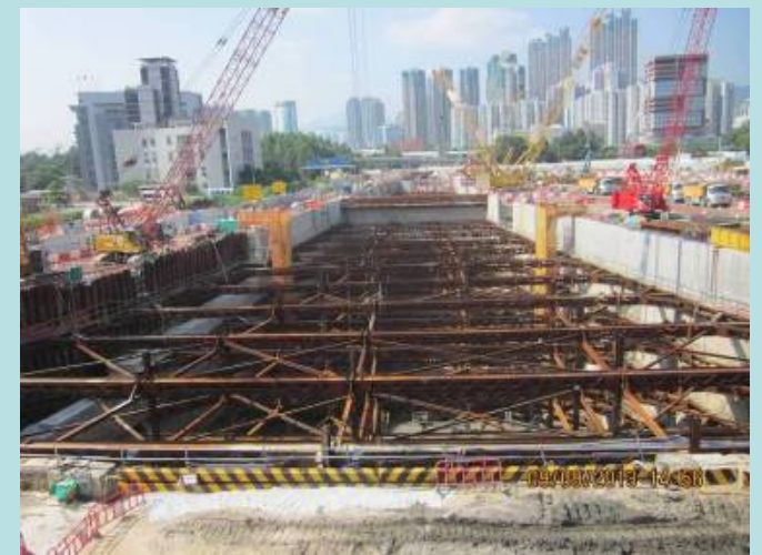
明挖隨填工程 Cut & Cover works
