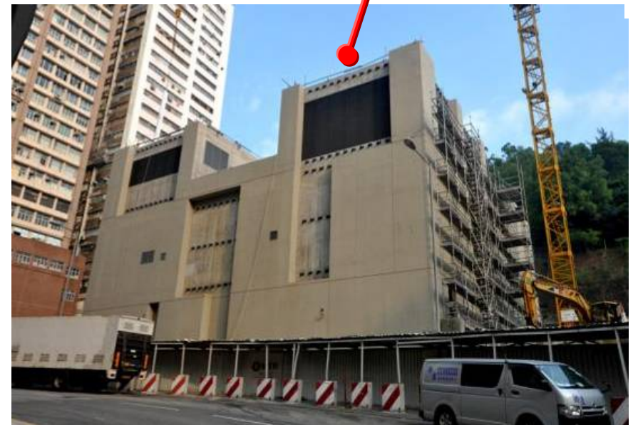
葵涌通風樓 Kwai Chung Ventilation Building
