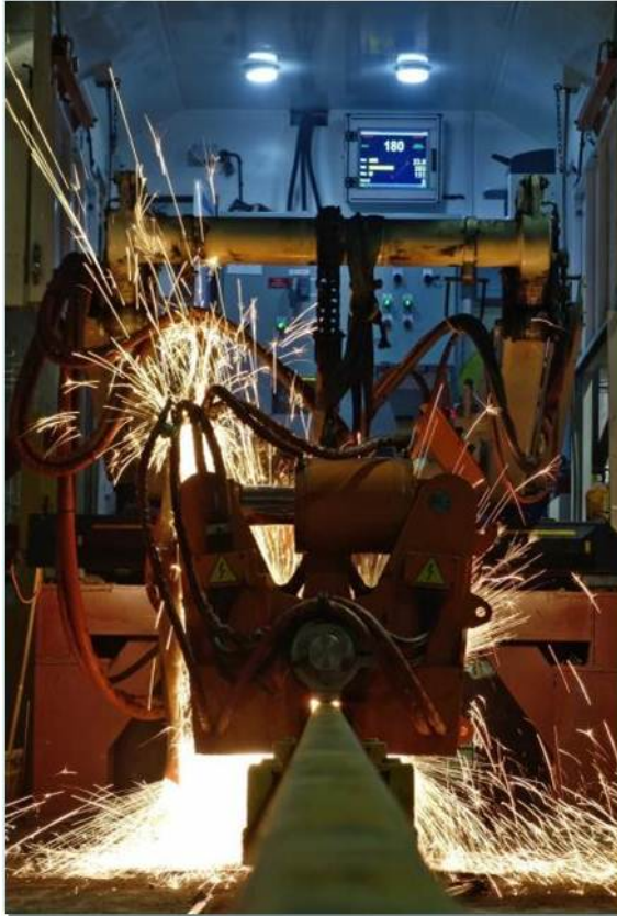
於路軌進行閃光電焊 Flash Butt Welding for Rails
