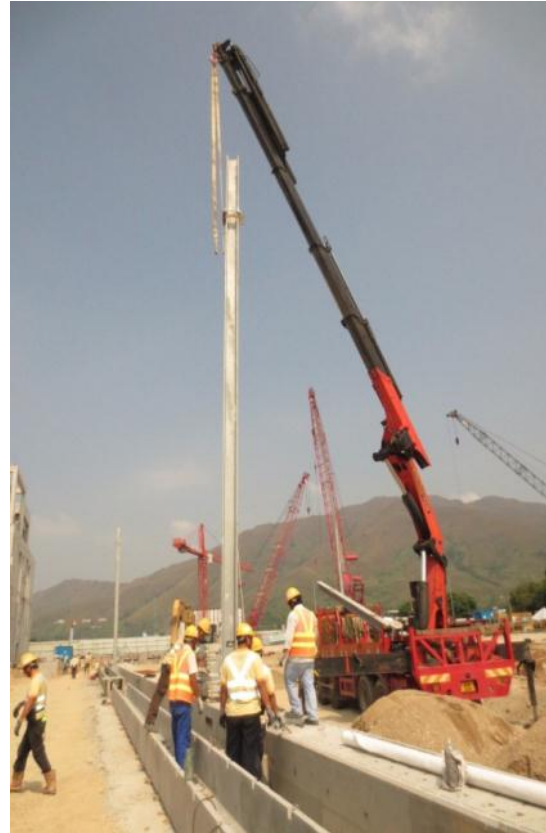
豎立高架接觸網支柱 Overhead Line Mast Erection
