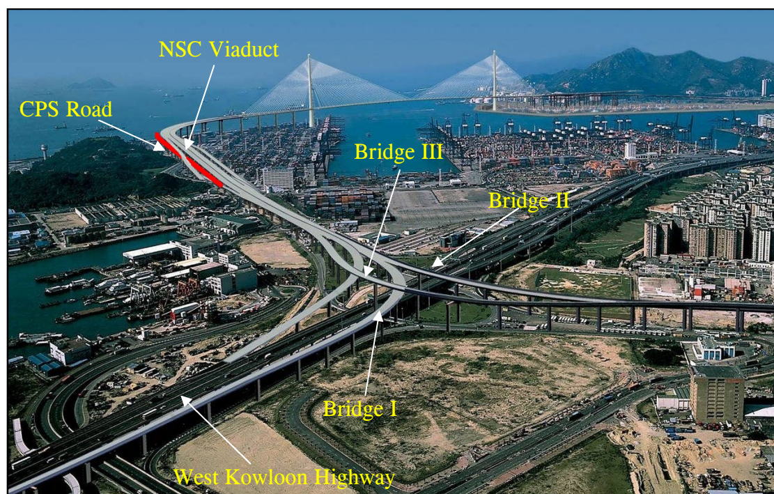
Bridges I, II and III
