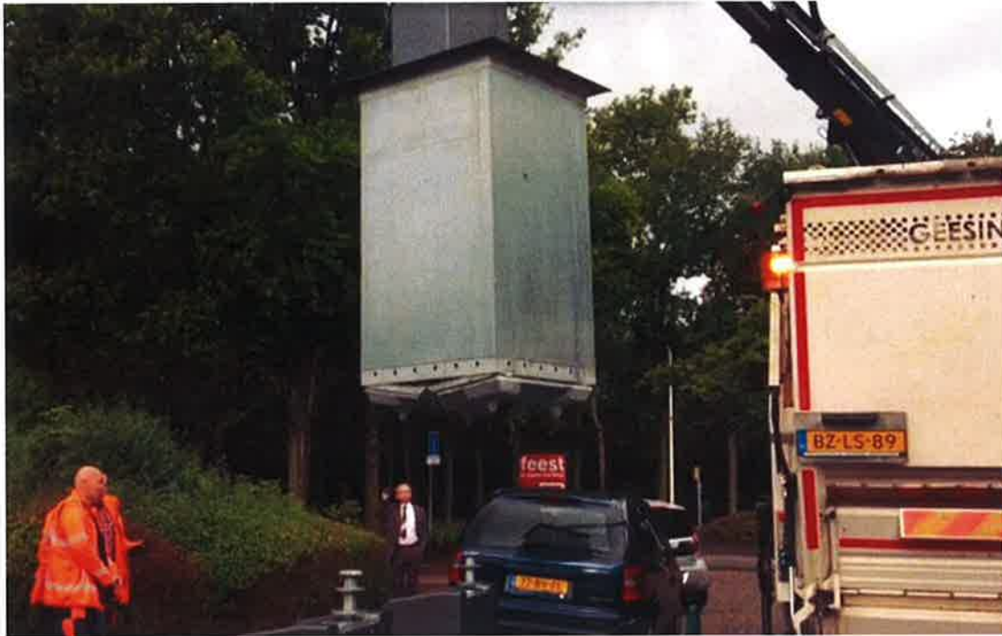
(WSS waste container being lifted out the ground)
