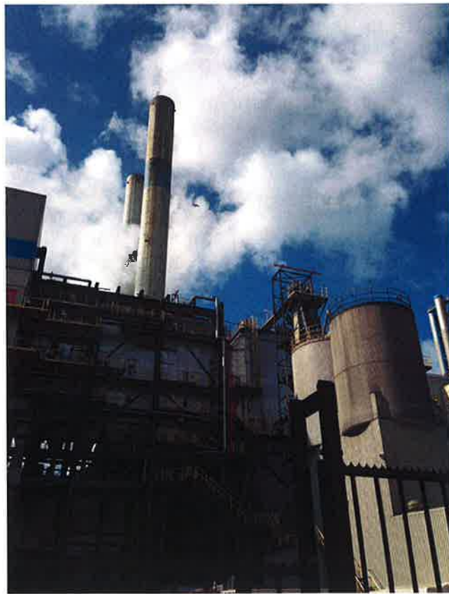
(RAV Incinerator chimney stack)
