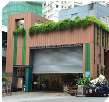
Current Refuse Collection Point in urban district
