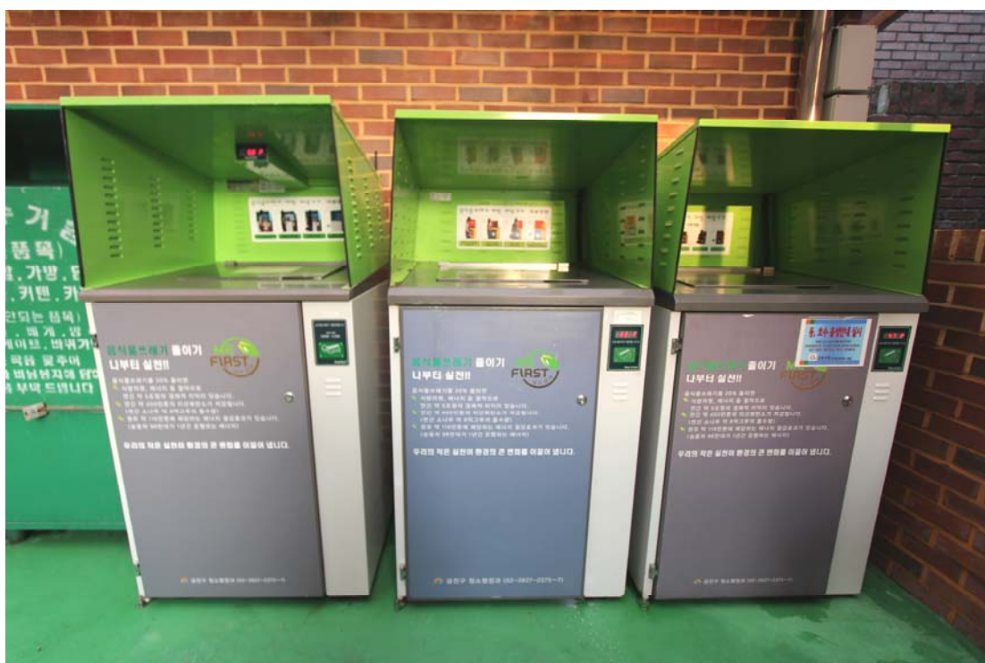
Collection bins installed with RFID chips to keep track of food waste generation by individual households
