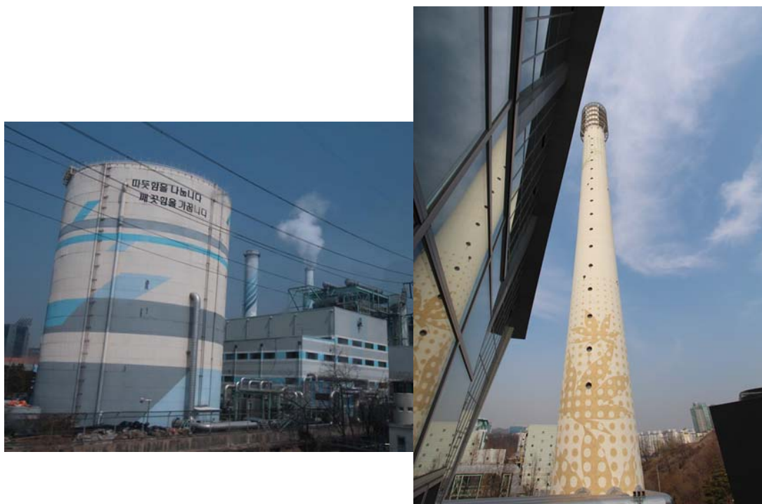
Emission of filtered gas from the stacks at the Mapo Resource Recovery Plant
