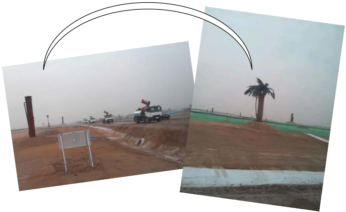
The landfill gas vents at the Sudokwon Landfill were disguised as trees ; trucks were spraying pesticide onto the Landfill
