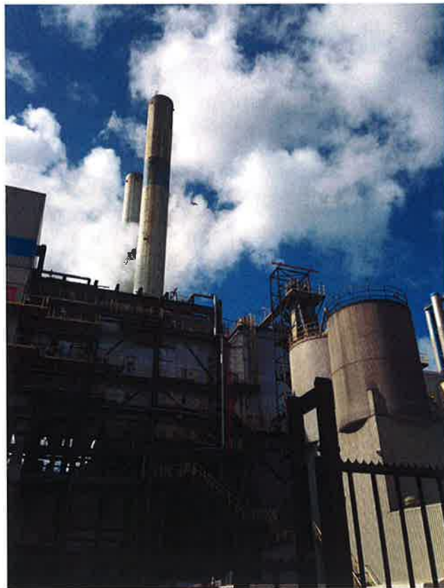
(RAV Incinerator chimney stack)
