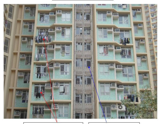
Tenants usually install laundry T-rods outside living room facade The pole holders at the re-entrant are left idle.
