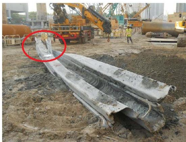
Deformed piles removed at Nam Cheong Station site.
