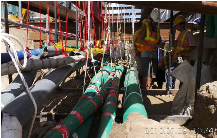
Excavation exposed complex and congested underground utilities beneath Jordan Road.
