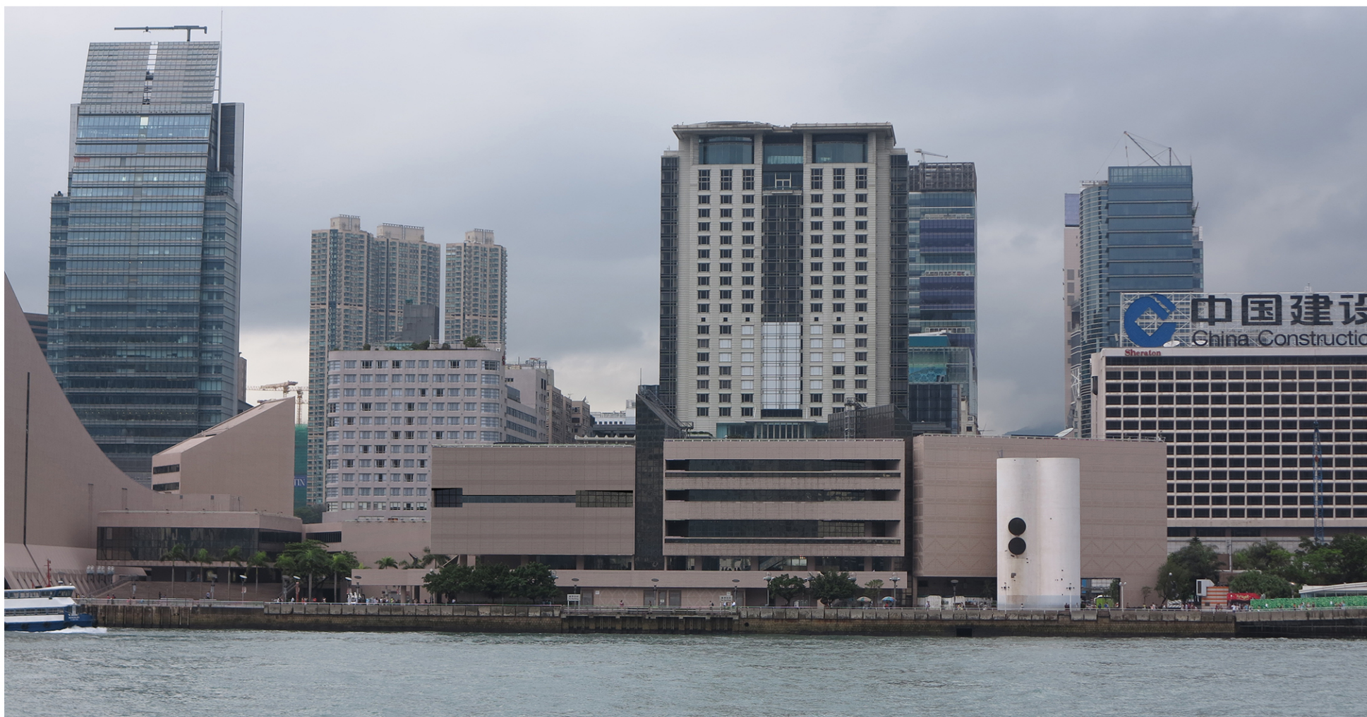
從南面望向藝術館的現貌照片 VIEW FROM SOUTHERN DIRECTION (SITE PHOTO OF EXISTING VIEW)
