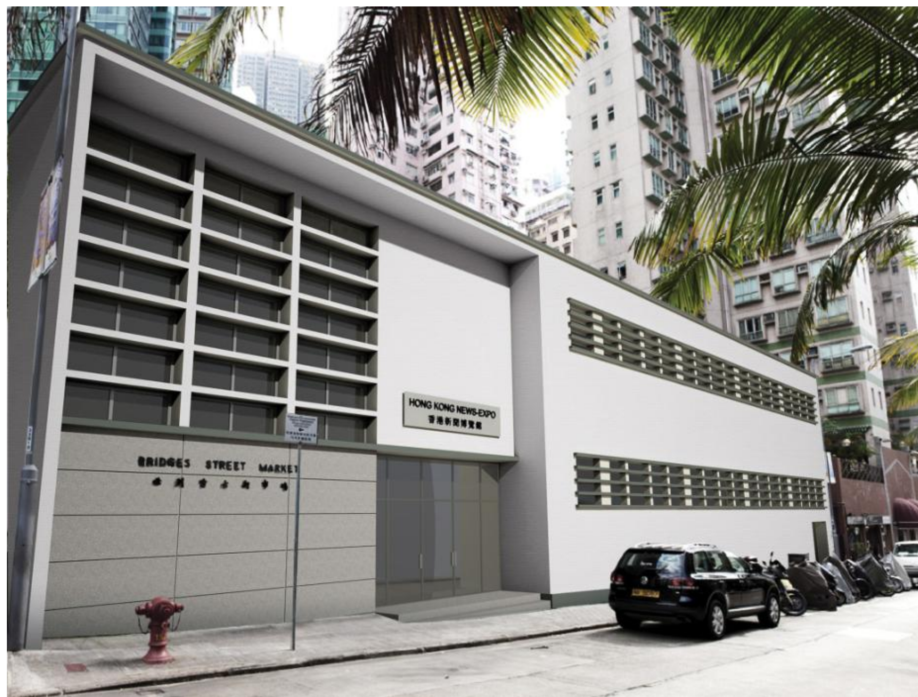
Looking from Bridges Street 從必列者士街的景觀
