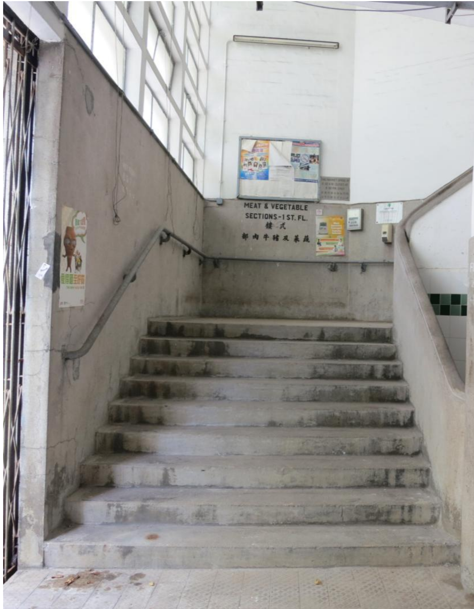
Staircase, shanghai plaster and stencil lettering 樓梯，上海批盪牆裙和傳統模版字
