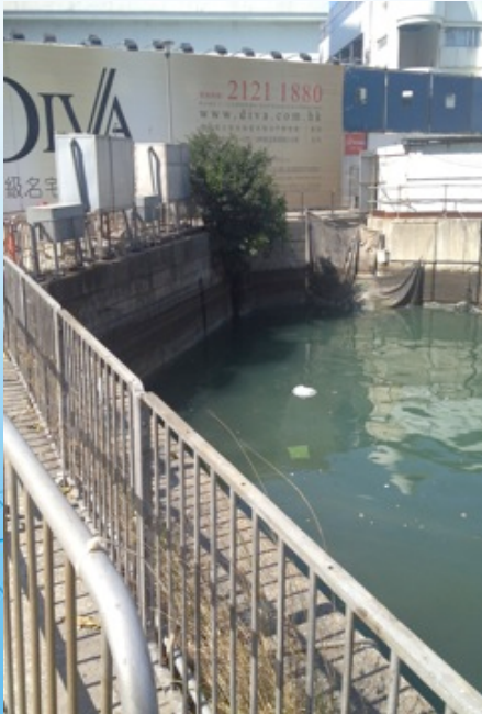
目視檢查和氣味巡邏 Visual inspection and odour patrol
